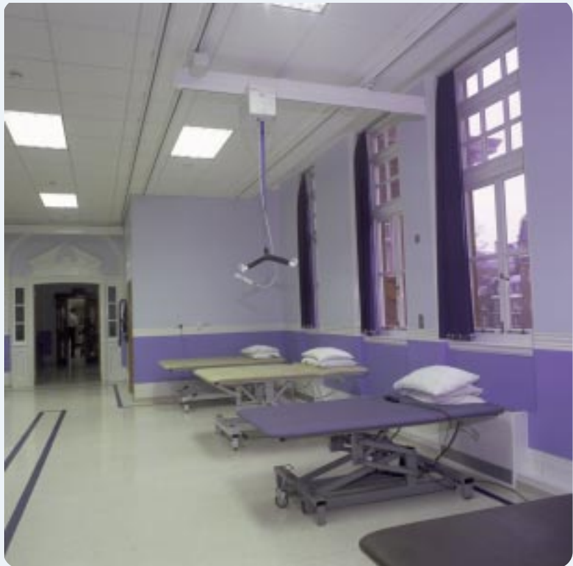
Two Wispa Ceiling Mounted Hoists provide complete room coverage on the hospital ward
