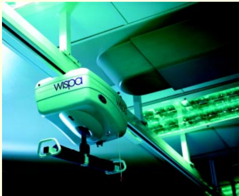
The Wispa hoist is carefully positioned in relation to the ceiling structure
